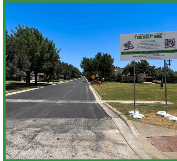
The entire section of roadway is receiving new paving, and striping improvements include a new center line as well as shoulders that can be used for parking or bicycles.
