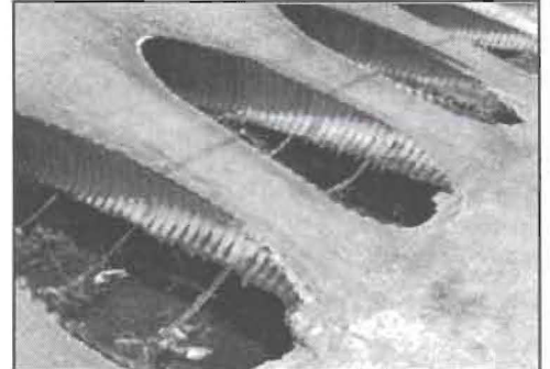
Mallard Lane drainage culverts that are rusted out.
