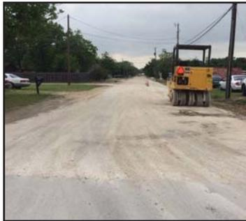
Reconstruction continues on 4th Street. To date, utility adjustments, relocation of pipes and lime stabilization on the eastern portion of the street are complete. The timeline has been revised for the relocation of shallow gas lines.
