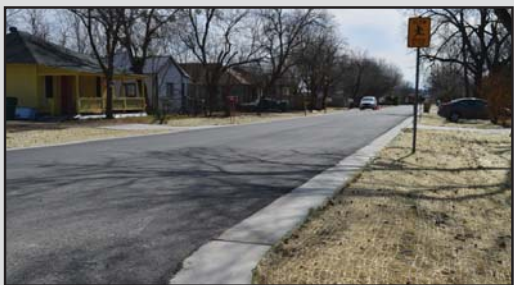
A look at newly rebuilt Edmond Street, facing south at 6th Street. It's open and ready for traffic. City Council, staff, citizens and contractors held a ribbon-cutting ceremony on site on February 8.
