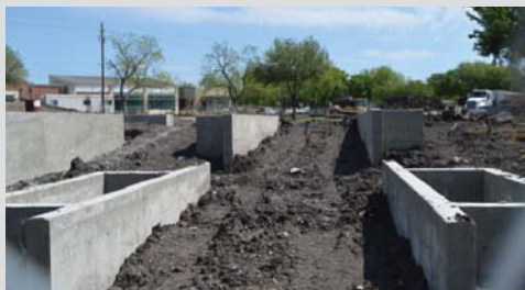
The new entrance takes shape at Heritage Park.
