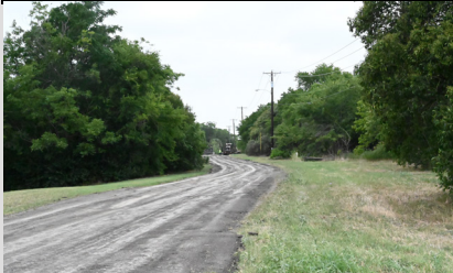
Public Works recently completed a level up to Gravel Pit road as part of the City's level up program.
