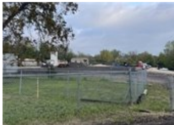
Construction recently began at the Taylor Animal Shelter.
