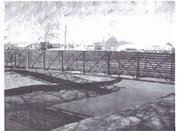
Hike & Bike bridge completed at Murphy Park
